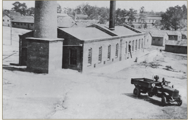
Hospital Boiler House (Building 160), c. 1919.
