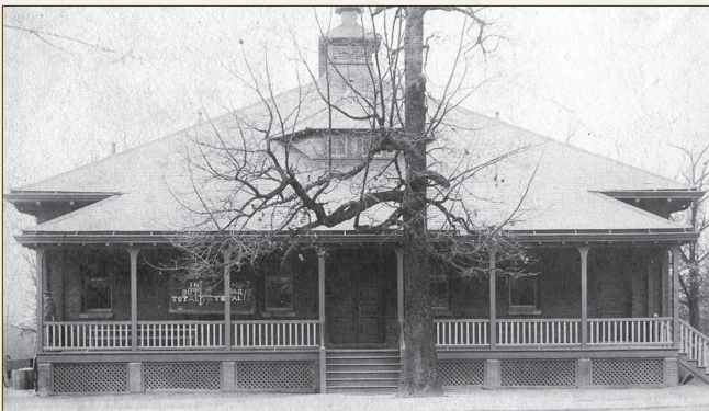
North Elevation of Post Guardhouse (Building 51), c. 1915.
