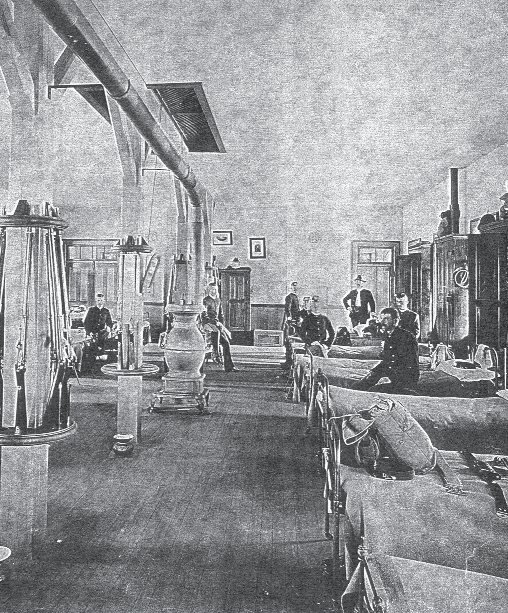
Interior of a Troop Row Barrack, 1893.
