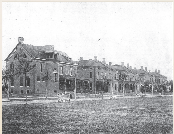
Staff Row Looking East (Buildings 5-1), c. 1893.
