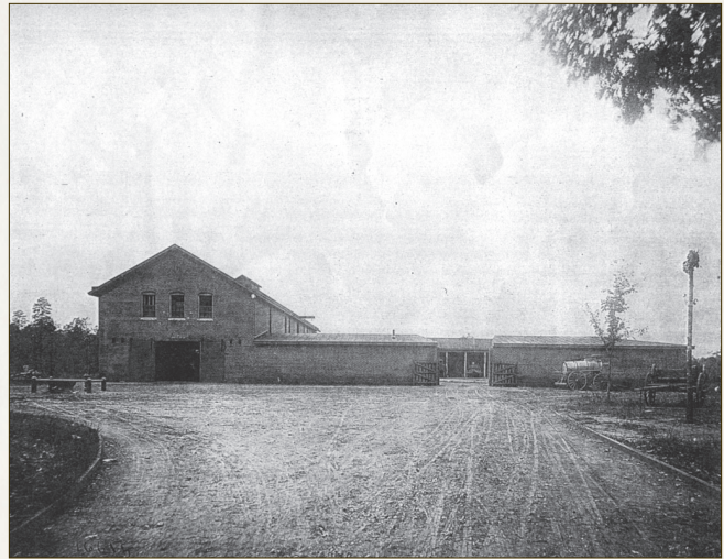
Quartermaster Stables (Building 400), c. 1892.
