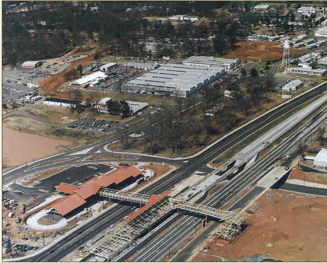
Construction of the Lakewood-Fort McPherson MARTA Station, 1984.
