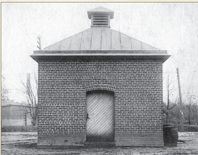
Oil House (Building 105), c. 1915.
