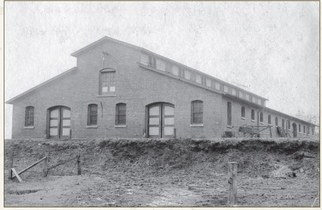
Quartermaster Stables (Building 401), c. 1915.
